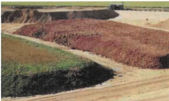
Clearly defined stockpiling of different soil materials
